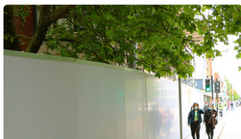
Secure & Sustainable Hoarding
